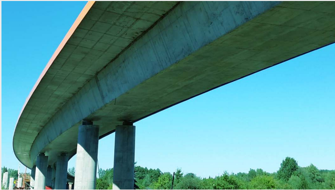
S7 expressway, part B: Ostróda Ring Road, part C1 Ostróda-Rychnowo (Poland) 210 pcs. of pot bearings with max vertical load 26000 kN 76 pcs. of elastomeric, guide and restraint bearings
