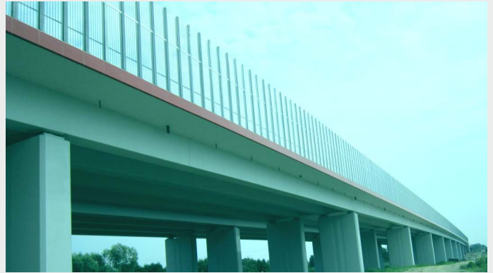
A4 highway from Tarnów to Rzeszów (Poland) 428 pcs. of pot bearings with max vertical load 13470 kN
