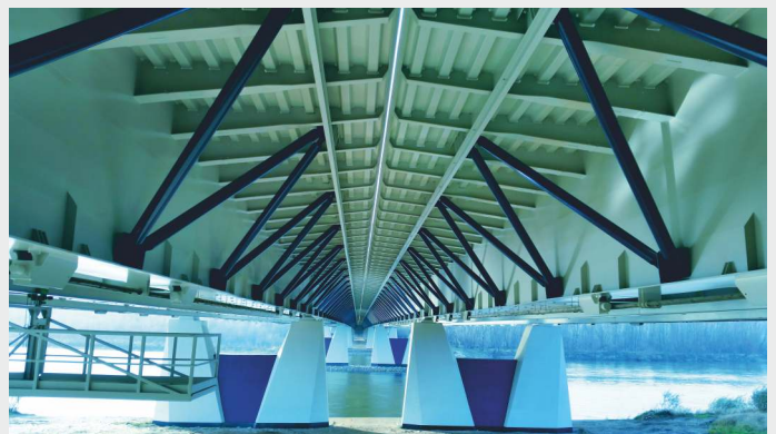
S8 expressway, Grota-Roweckiego Bridge, Warsaw (Poland) 32 pcs. of pot bearings with max vertical load 27400 kN 32 pcs. of elastomeric, guide and restraint bearings
