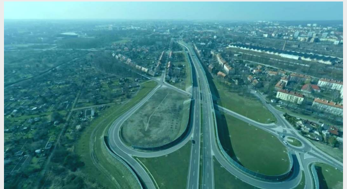
Central expressway, Gliwice (Poland) B2W joints with movement from \pm 40\text{ mm} to \pm 200\text{ mm}
