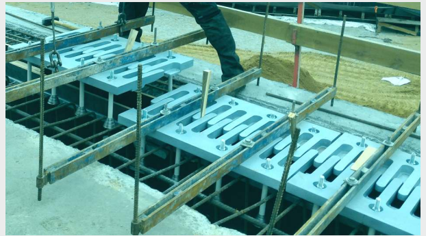
Picture 16. Preliminary installation
