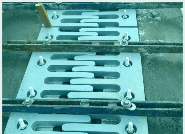
Picture 16. Concreting the recess
