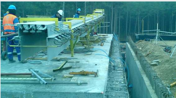
Picture 12. Installation of modular expansion joint
