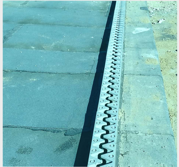
Picture 14. Single-seal expansion joint after installation
