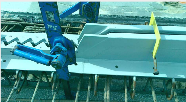
Picture 13. Installation of single-seal expansion joint
