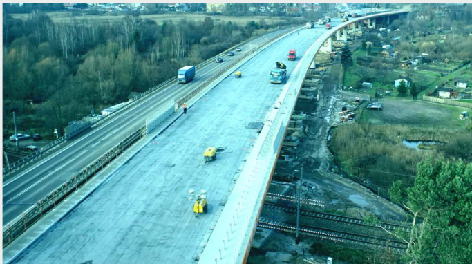
S7 expressway, Ostróda Ring Road (Poland) B2P joints with movement from \pm 150\text{ mm} to \pm 200\text{ mm} B2NN joints with movement \pm 100\text{ mm}
